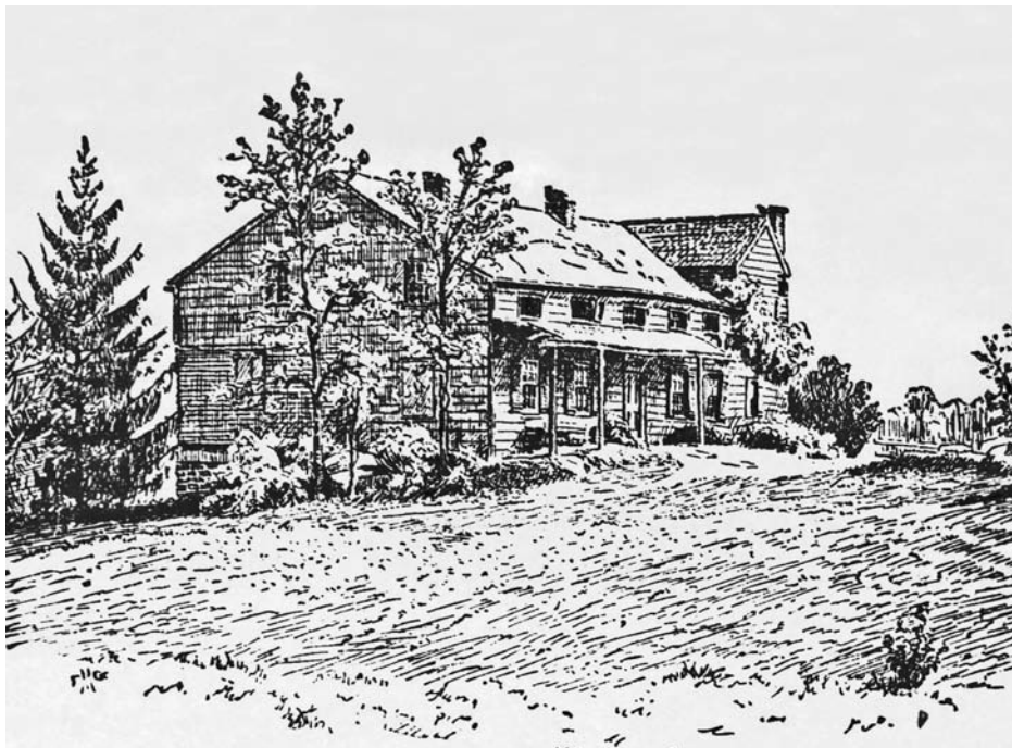
Charles Guion's Tavern was popular during the colonial and revolutionary era. During the war, General George Washington was a guest. Rebecca Turner, a former slave, was a well known as a tavern cook. The building burned down in 1909. When the masonry walls were pulled down, a large number of gold coins were found.
