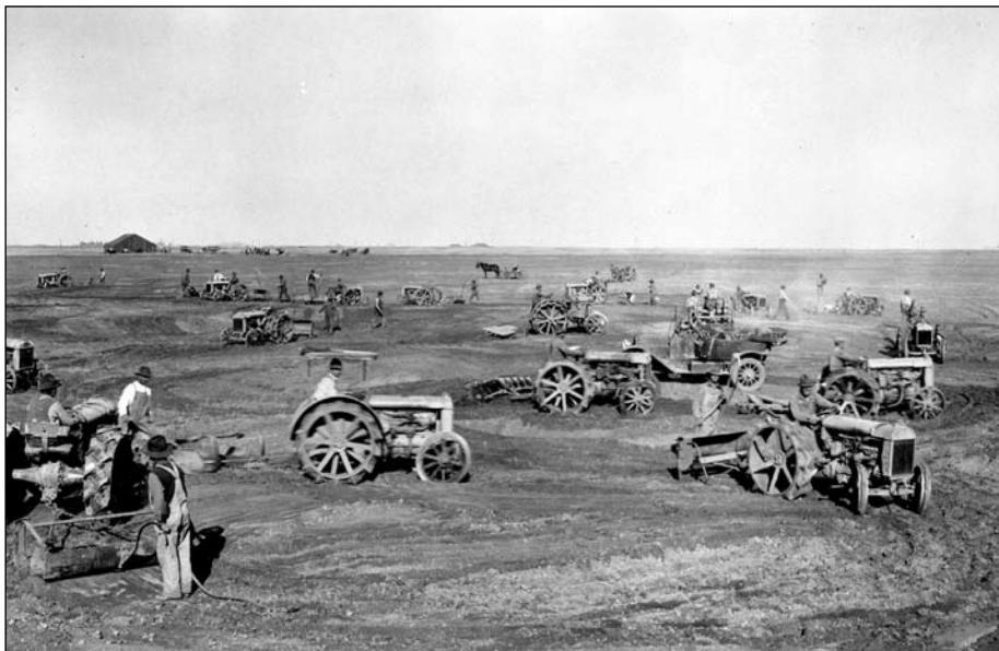
Leveling the land with "motorized" tractors.
